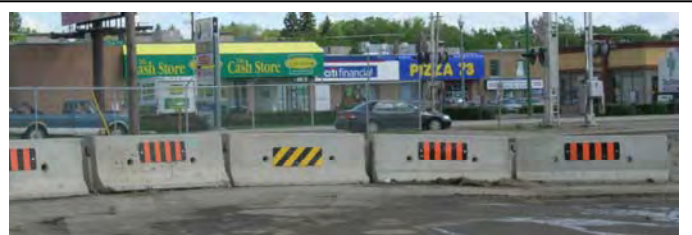
Traffic barricades on Avenue G and the CPR ROW
